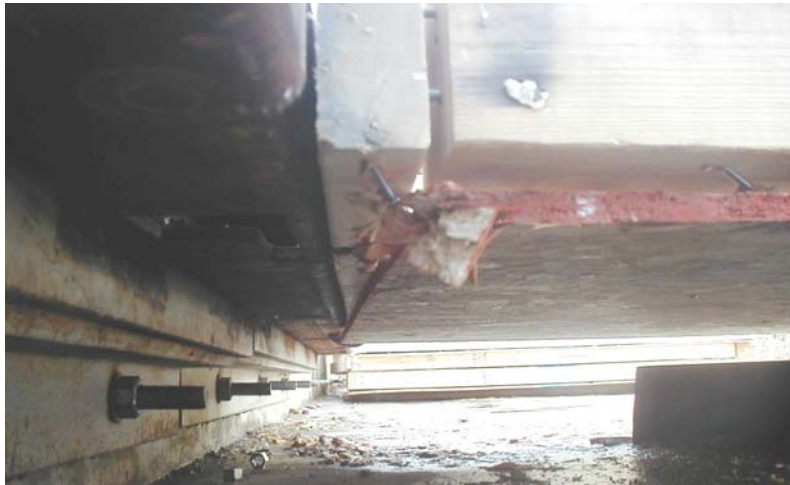
Figure 17: Unzipping of nails on bottom plate (OSB)
