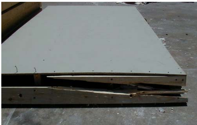
Figure 58: Bottom plate splitting parallel to grain
